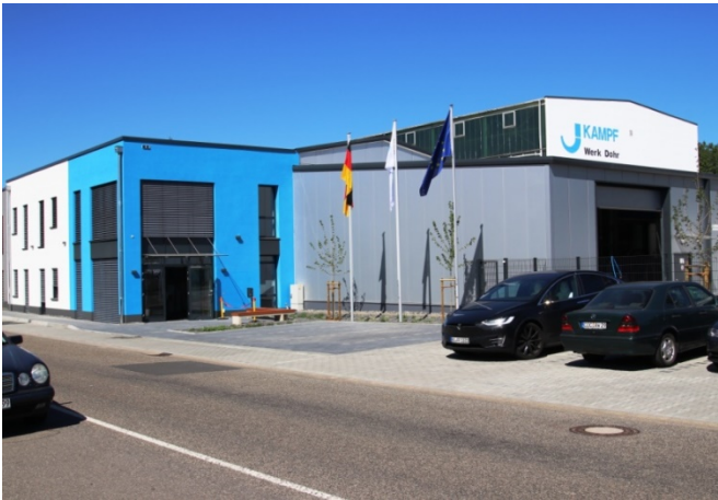
The new administration building at Dohr.
